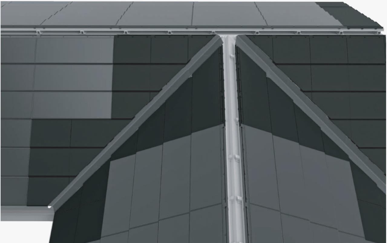
Auxiliary tile installation completed
